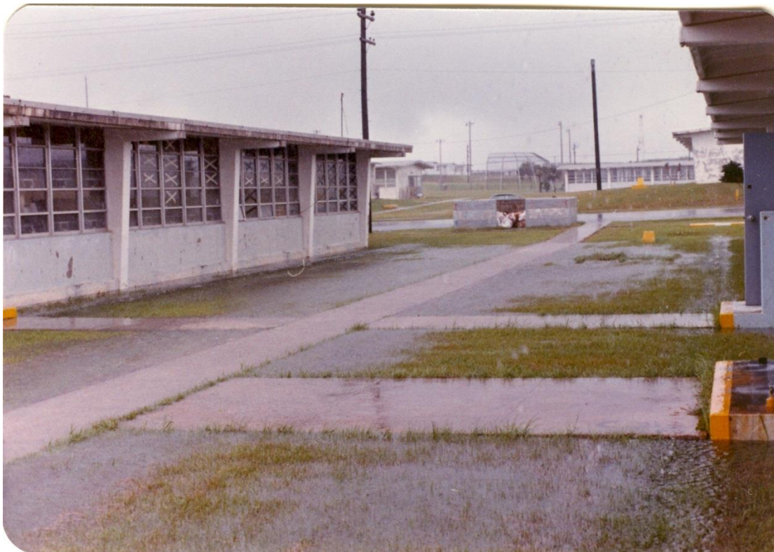
It could rain in Okinawa, parts of days often looked like this though this was a Typhoon downgraded to a Tropical Storm. The X's on the windows are tape in preparation for a pending Typhoon.
